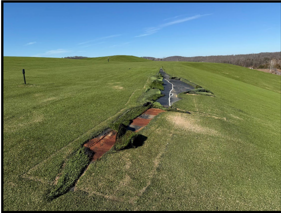
Photograph 11: View of DCT-4 on east side of Area 1-3, above LCS-7 near 36.459656, -92.445638.
