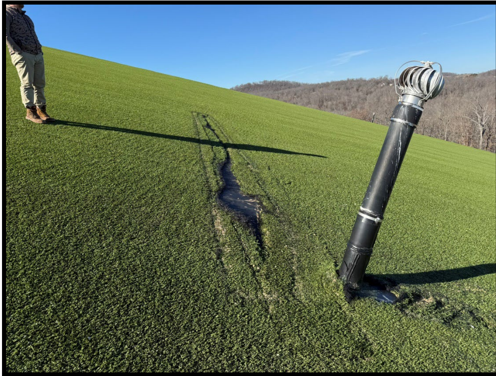
Photograph 5: View of DCT-1 on north side of Area 1-2, at 36.46181, -92.45045.
