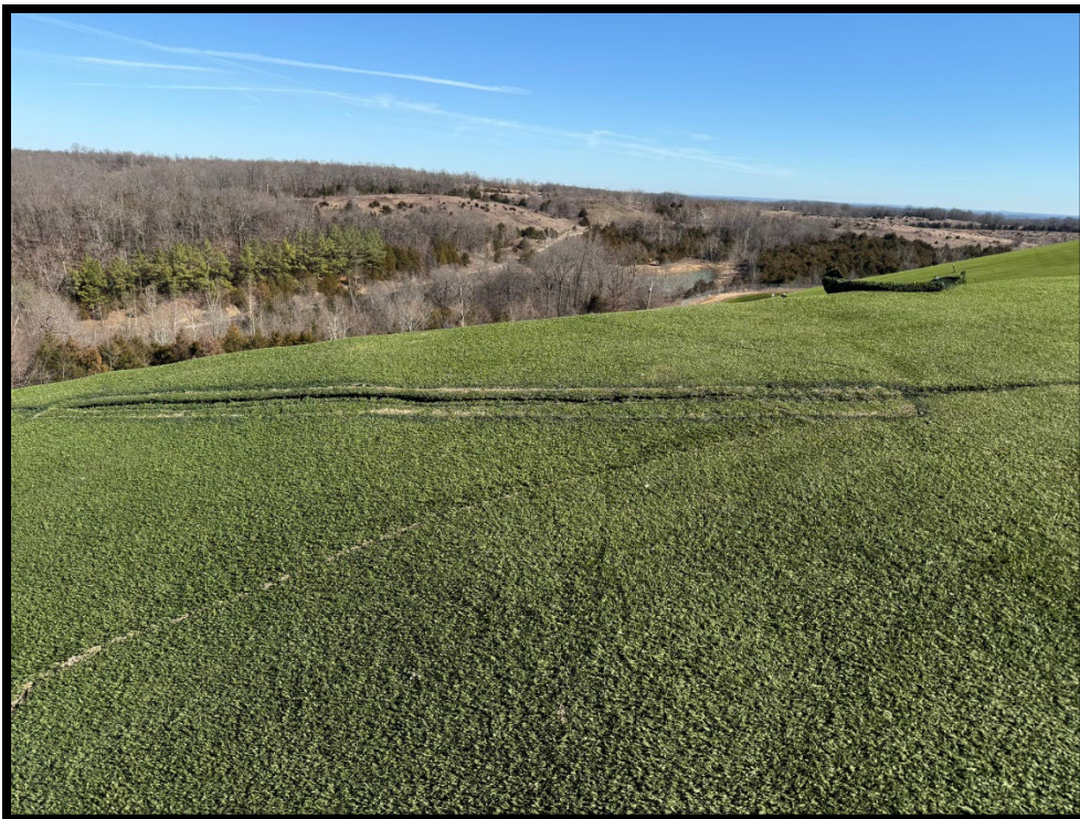
Photograph 8: View of DCT-2 on top of north side of Area 1-2, near 36.461453, -92.450493.
