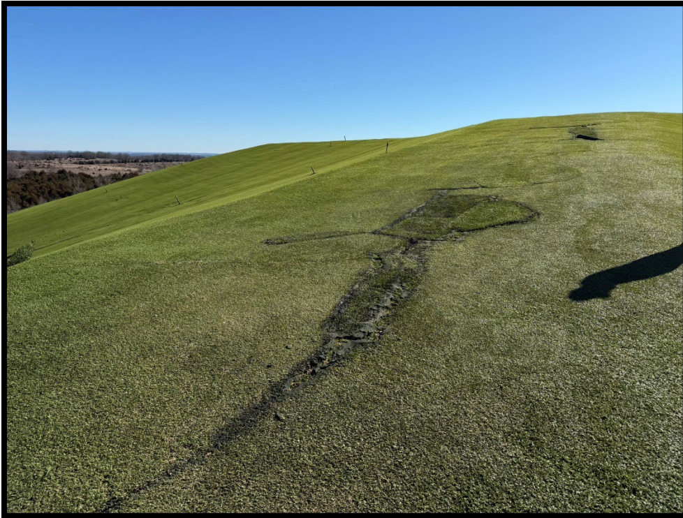
Photograph 7: View of DCT-2 on top of north side of Area 1-2, near 36.461453, -92.450493.
